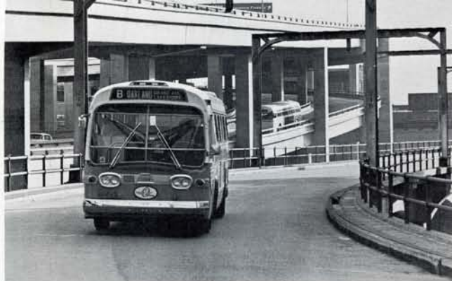
Coming into San Francisco off the Bay Bridge, coaches travel to the terminal on their own exclusive road.
