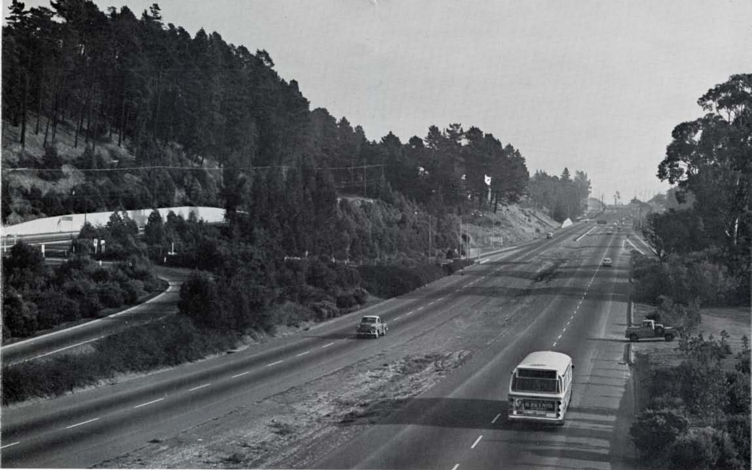
Expanding freeway construction has made possible faster schedule speeds, and helped make a success of new express service.
