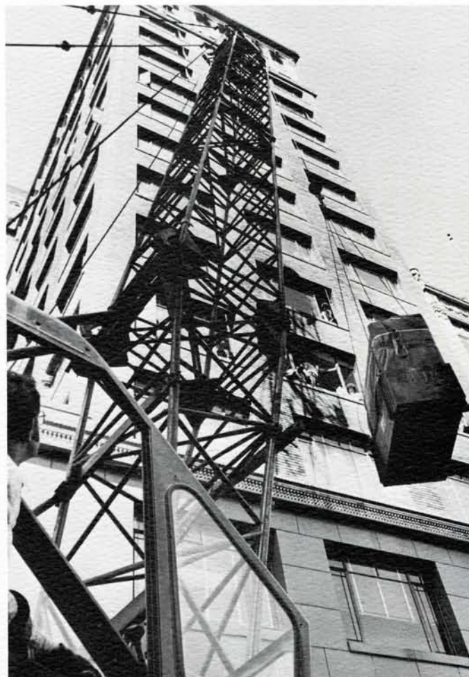
A ton of computer soared four floors above the streets of downtown Oakland. District offices received a new IBM 360/30 computer the hard way — removing window glass first — to better Data Processing capacity and programming flexibility.
