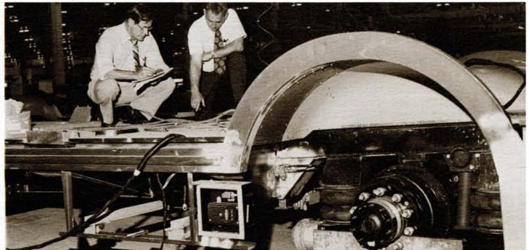
Assembly of 120 new Flexible coaches proceeds under watchful eyes of Maintenance Manager Anthony R. Lucchesi, left, and Maintenance Superintendent Glenn A. Ashmore. Buses were first off new assembly line.
