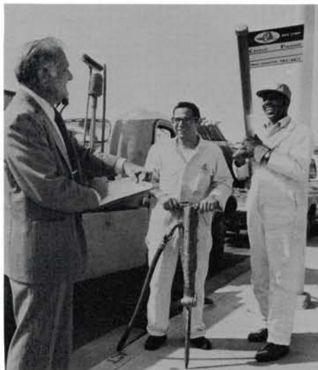
Fremont city traffic engineer Myron Harmon checks list of bus stop sign locations as George P. Spinella, center, and Lonnie L. Kelly right, prepare to make an installation.
