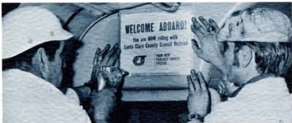
Maintenance worker Wayne West, left, from AC Transit, and Michael Lang, of Santa Clara County Transit District, work together installing car card in a San Jose bus. AC Transit helped the new district get into operation under a unique management contract.
