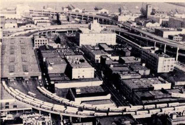
Buses stand ready at Transbay Transit Terminal to carry over half of people now using Bay Bridge in travel peak.
