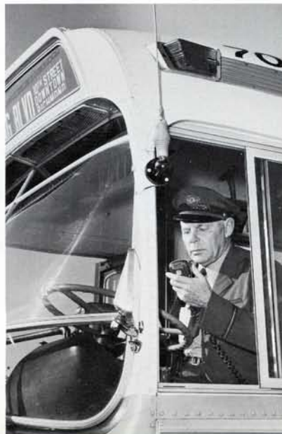
Operator makes test call with two-way radio to check effectiveness of planned communication network.
