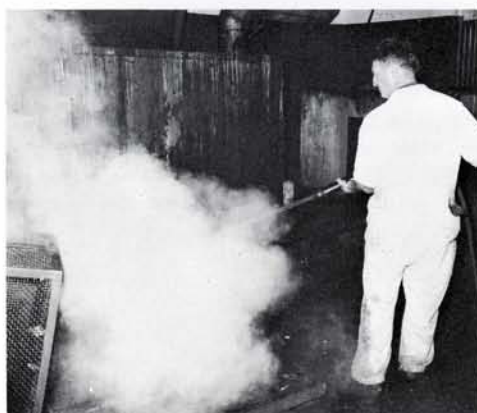
Engine parts receive thorough steam cleaning before they are reassembled during major bus overhaul.
