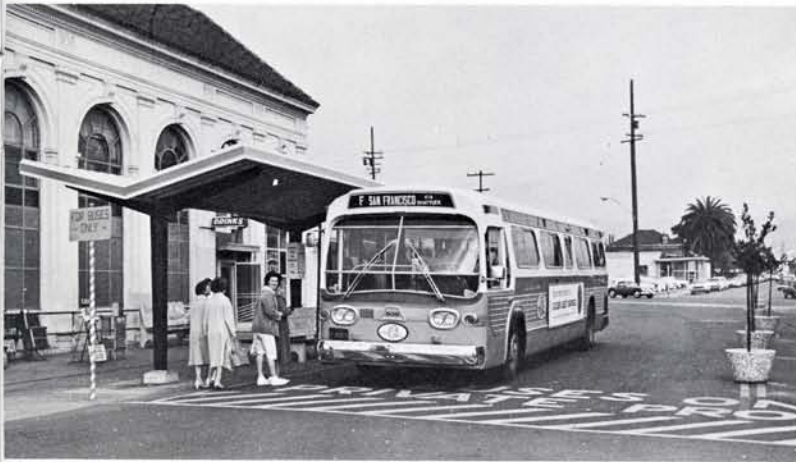
New modernistic shelter is installed at San Pablo Station—one of East Bay's oldest and best known transfer points.
