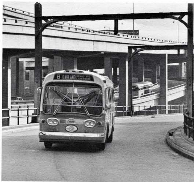
Buses travel from Bay Bridge into Transbay Transit Terminal in San Francisco on exclusive elevated roadway.
